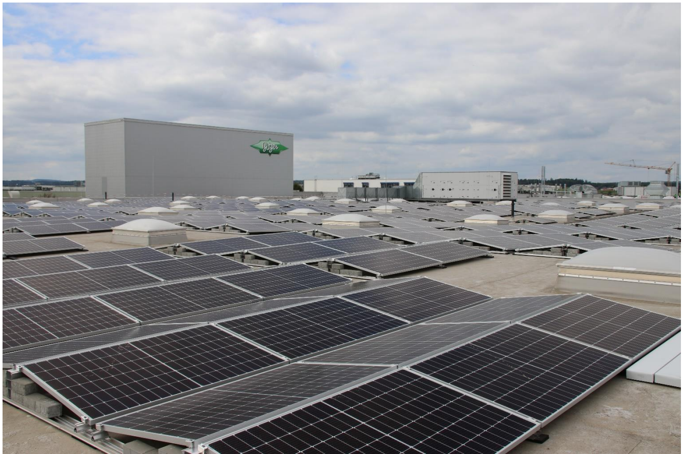
Image 2: Sustainability is a topic of concern for today's job applicants. At the BITZER production site in Rottenburg-Ergenzingen, solar panels generate over 60 per cent of the electricity required for operation
