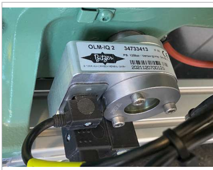
Fig. 44: Oil level controller OLM-IQ2 (part no. 347 334 13) at the compressor (example)
